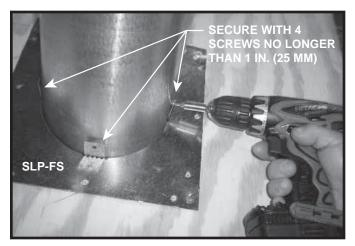
Figure 10.18 Secure Pipe with SLP-FS
